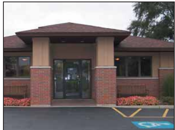
Fig. 6 Rear building extension adjacent to drop-off lane in parking area.
