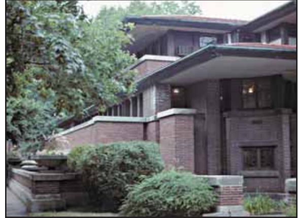
Fig. 2 Wright's Robie House in Chicago. (Photograph by Jeffery Howe.)
